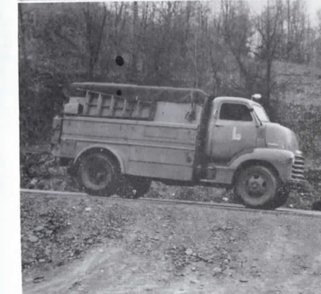
At top the Bradley station in construction, in center a new transformer for Bradley, at bottom one of the many service trucks.
