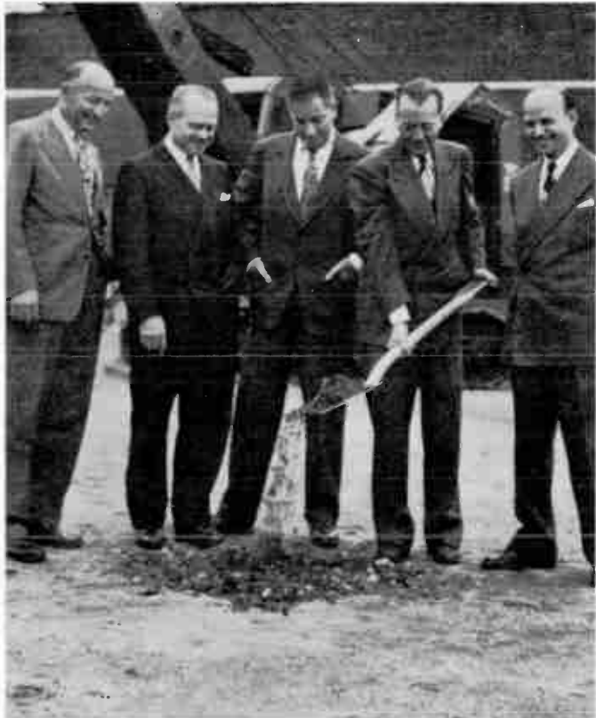
7 NEW ERA: Under the ownership of The Philadelphia Inquirer, WFIL is constantly expanding its facilities. At the ground-breaking for a new television studio building, Louis E. Littlejohn, Chief Engineer; Roger W. Clipp, General Manager; Walter H. Annenberg, Publisher of The Inquirer; Kenneth W. Stowman, Television Director, and Joseph A. First, Inquirer Vice President, officiate.
