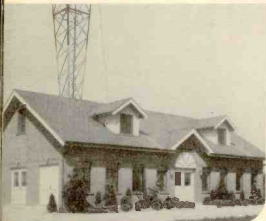
This building houses the transmitting equipment of WBNS. Thousands of dollars of the best radio equipment in the country is operated from this point to give Central Ohio the best radio reception.
