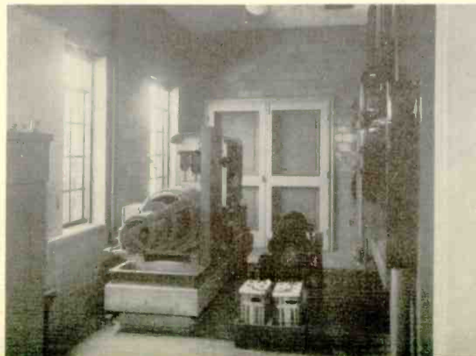
The generator room at the WBNS Transmitter. The large generator to the left is the 25,000 watt auxiliary power plant, driven by a Ford V-8 motor, and whereby WBNS may generate its own power for days in an emergency. This is the only radio station in Central Ohio so equipped.
