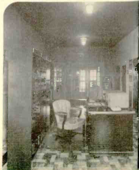
Control Desk, Measuring and Test Equipment. On the desk is the console where music from the studios is controlled and monitored before going into the transmitter. This console also provides facilities by which WBNS may run programs from the transmitter in emergency, and for testing purposes. The rack contains test and measurement equipment by which the transmitter equipment is maintained at the highest point of efficiency by daily and weekly tests.
