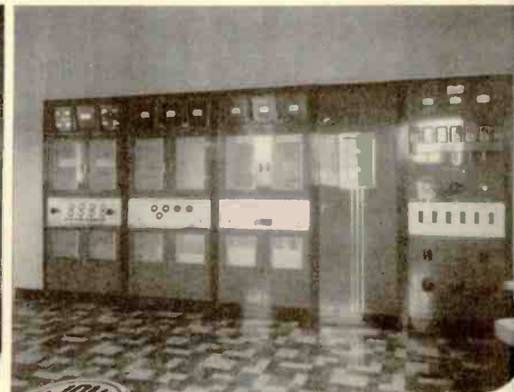
The regular WBNS 5000 watt Transmitter, the very last word in equipment, installed in the spring of 1938. Automatic circuits incorporated in this transmitter are too numerous to mention and make possible switching so rapid that the listener is unable to detect the operations. The use of air-cooled tubes, three of which are 5000 watters, replace the former water-cooled type. WBNS was the first high powered station to make this modernization.
