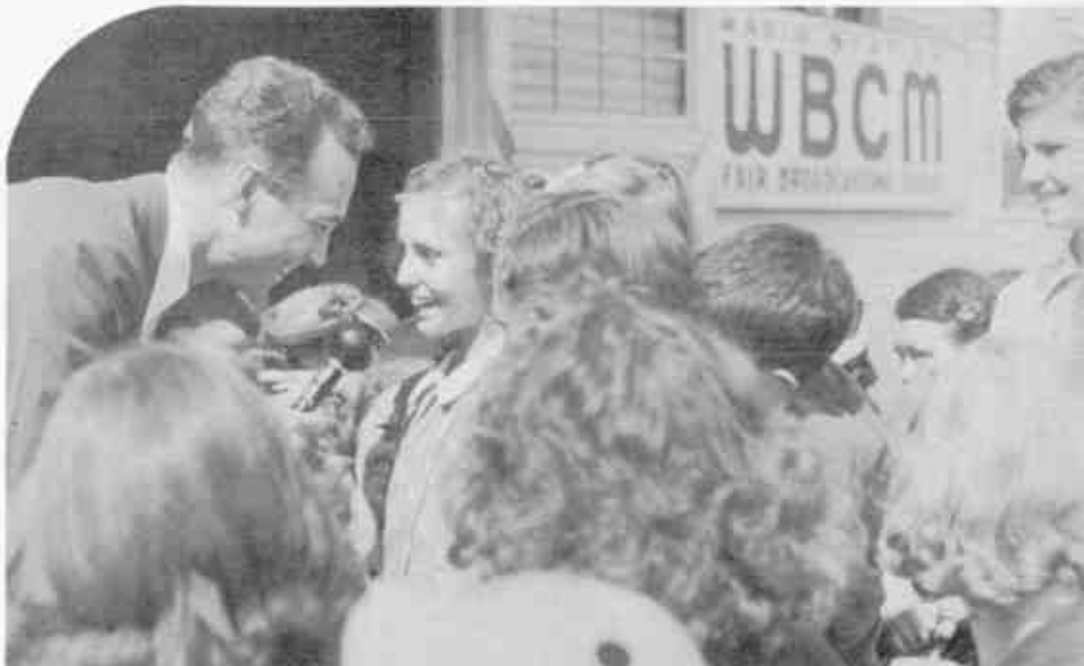
Behind All WBCM "Special Events" is the remote-control staff of WBCM engineers. Chief Engineer Ralph Carpenter is shown here with the portable amplifier, at the Ridotto fire. Microphone lines lead into the amplifier before him, where volume is regulated and additional electrical current is applied to "boost" the sound to the transmitter.
