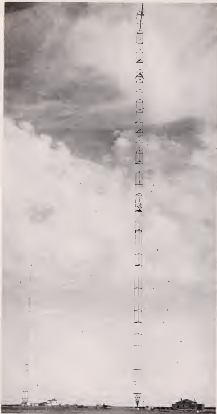
Here's the new 915-foot tower of WKY, Oklahoma City, which will go in operation late Summer or early Fall. When the 90-foot FM aerial is perched atop the huge AM tower, this will be the tallest mast in the U.S.A. Transmitter equipment and grounds represent a $250,000 investment.
