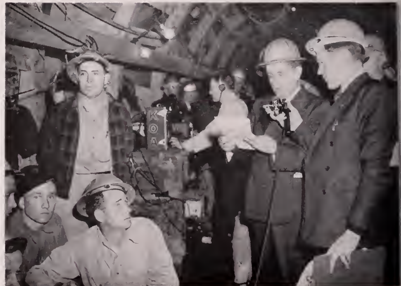
Ceremonies attending the historic "holing-through" of the Alva B. Adams diversion tunnel of the Colorado-Big Thompson Rivers project, were broadcast by KOA (Denver) from the heart of the Rocky Mountains. After four years of digging, a dynamite blast ripped out the last eight feet of granite that separated the east and west bores of the tunnel deep beneath the Continental Divide.
