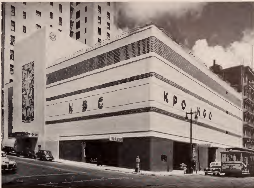
This modern NBC studio structure, recently opened in San Francisco, incorporates many architectural and engineering advances supervised by O. B. Hanson, NBC Vice-President and Chief Engineer. Golden Gate City's network shows originate here.
