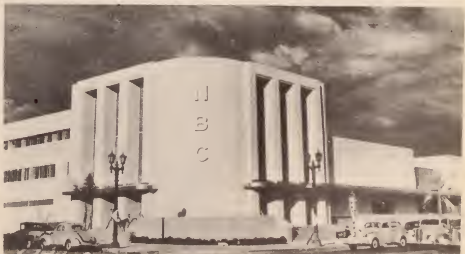
This is a view of NBC's new Radio City in Hollywood, looking north from Sunset Boulevard along Vine Street, showing part of the 300-foot terrace as it completes a graceful curve at the lobby. Part of the structure in the background is the three-story office building.
