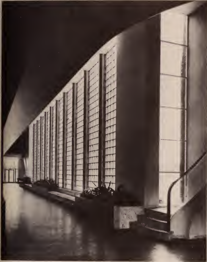
The Main Entrance Hall, 152 feet long, 14 feet deep and 23 feet high, on one side of which looms a high wall of glass blocks and on the opposite are separate entrances to five studios.
