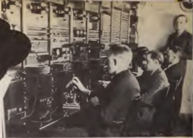
• MASTER CONTROL ROOM when W.E.A.F.'S headquarters were at 195 Broadway.
