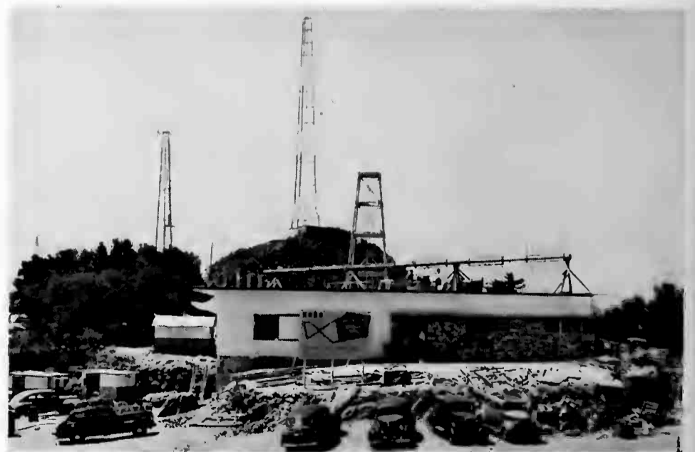
KNBH, the new NBC Television Station on Mount Wilson, Cal., nears completion. According to Raymond Guy, Manager of Radio & Allocations Engineering, KNBH will be conducting test operations by the middle of this month. From this spot over a mile high, one can see 100 miles on a clear day, with Los Angeles spread below in a vast panorama.
