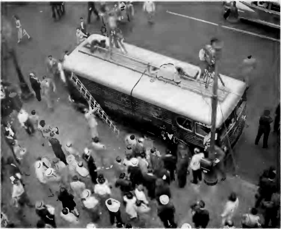
Truck and crew on location in Times Square. Jack Irving setting up ladder, on left. Note line on pole for telephone communication.
