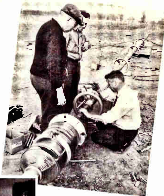
Engineers make final adjustments on the 4-bay FM antenna before it was hoisted to the top of the tall KFMX tower.
