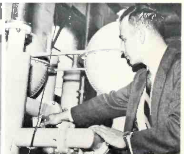
FILTER Victor Bary, NBC engineer who is helping to install KPTV's equipment, examines ultra high frequency filterplexer, which co-ordinates TV sound and image. Test pattern shown had "excellent" signal Thursday.
