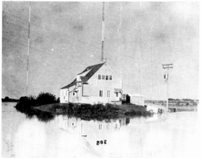
Not since June, 1947 have the KMA towers been surrounded by flood waters as they were this fall. When the unusual fall flooding of the Nishnabotna River occurred, KMA engineers, Chief Don Burrichter, Ralph Lund and Norm Kling, continued with their duties by rowing in from the highway in the boat, shown "beached" on the right side of the picture.
