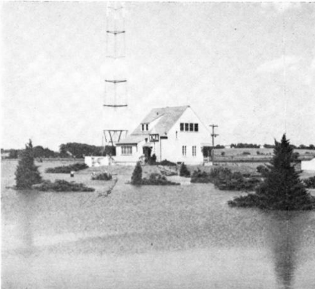
Flood waters have surrounded the Transmitter Building many times. One of the worst was in June, 1947 when this picture was taken.
