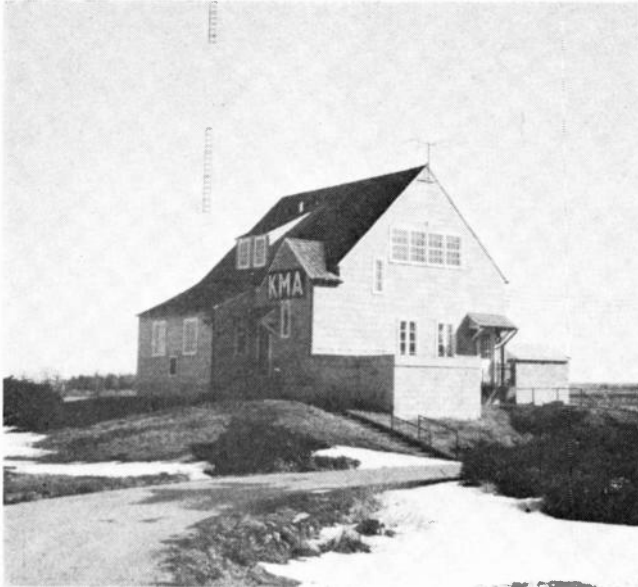
KMA Transmitter Building as it looks today after several additions. Improved tiling has helped the land's drainage problem.
