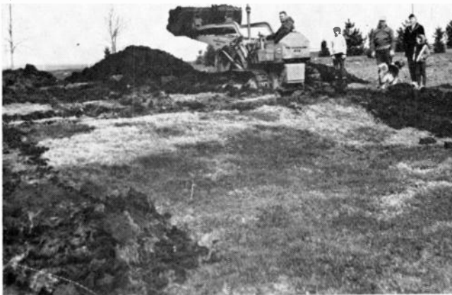
Excavation begins for new Gowing farm home.
