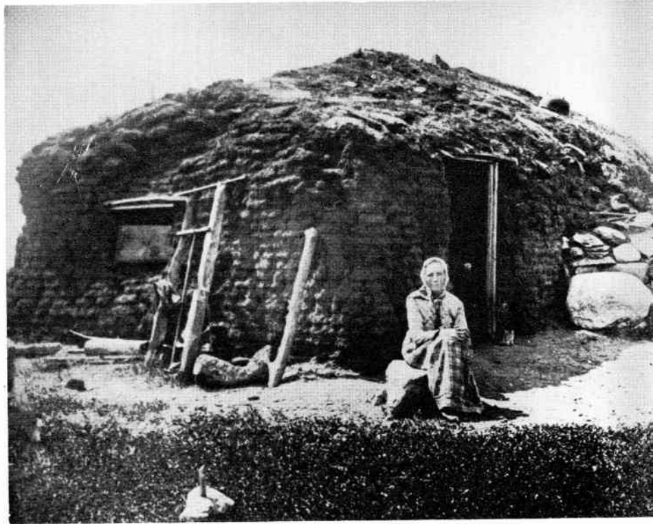
No housing shortage in the days of Minnesota's settlement as long as the good earth produced an abundance of sod. Houses such as this dotted the prairie sections.
