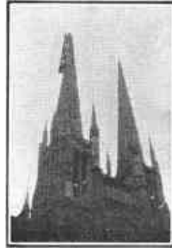
Bordeaux Cathedral, December, 1914, showing reinforced steeple to support radio antenna.
