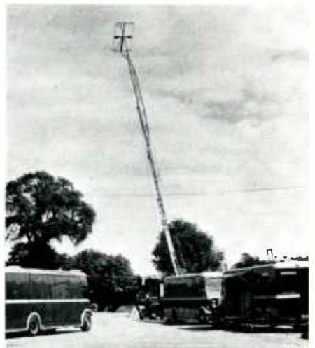
B.B.C. mobile television unit. The antenna raised on an extension ladder.
