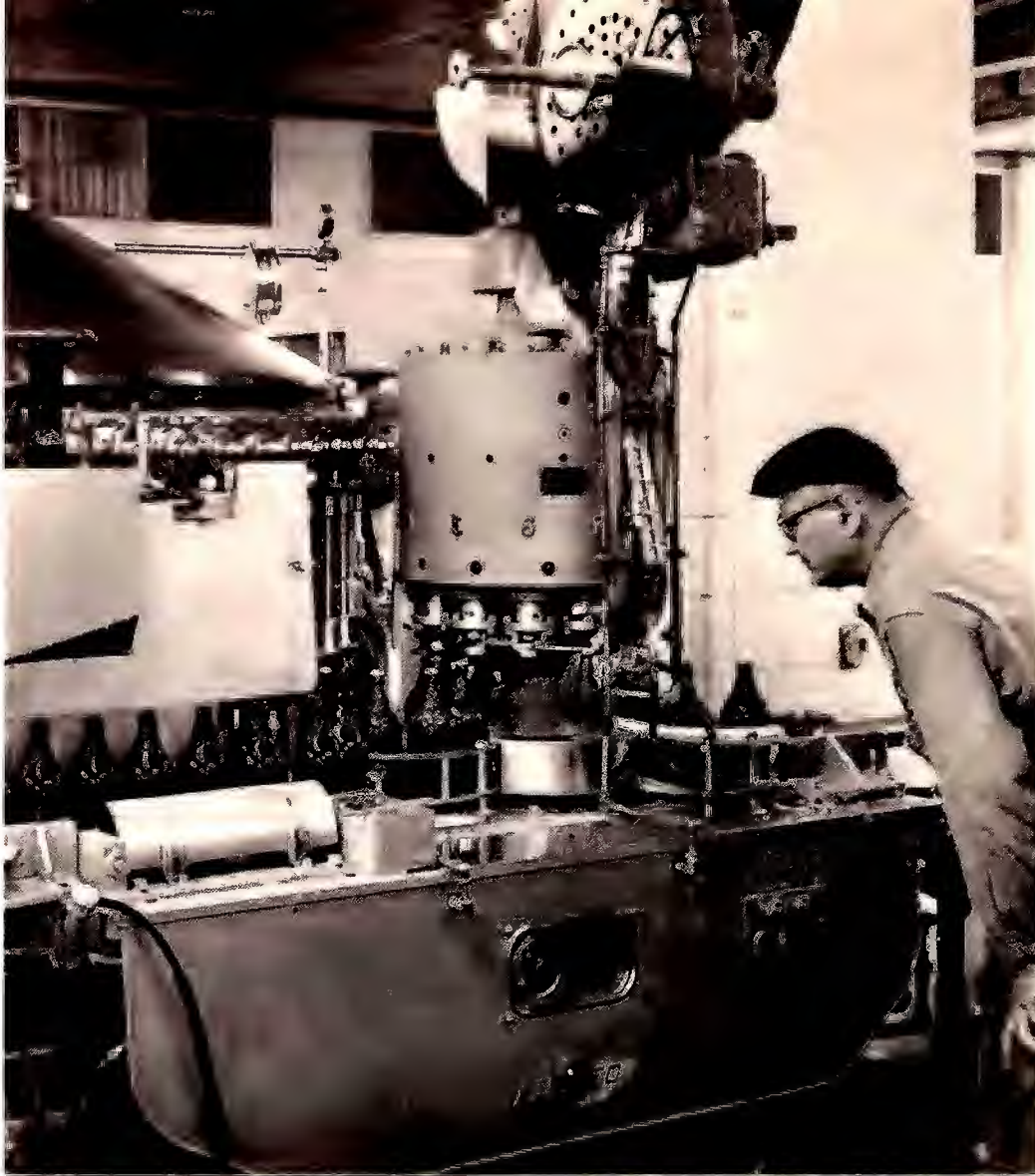
Bottling unit puts caps on 300 quart bottles per minute.
