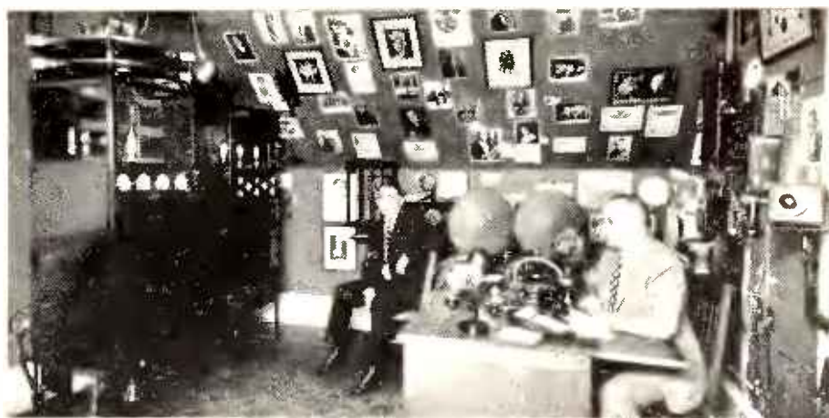
THE CONTRAPTION IN THE CORNER was "a mighty 20-watt transmitter with two switch panels, the power control panel containing four meters for the proper regulation of power and the second, the transmitter panel. Generators were remotely controlled."
