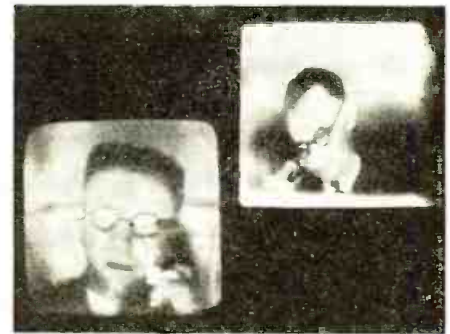
Above—Actual reproductions of the television images of two persons telephoning to each other, as observed on the monitor in the telephone exchange.
