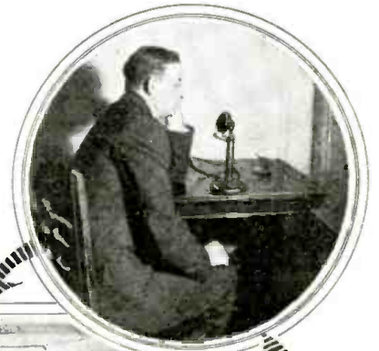
Left—Typical phone transmitter aboard 21 ships now sailing the Atlantic and fitted for carrying on radio phone traffic with subscribers on land. This transmitter is that aboard the S.S. “Empress of Britain.” Receiver below on “De France”.
