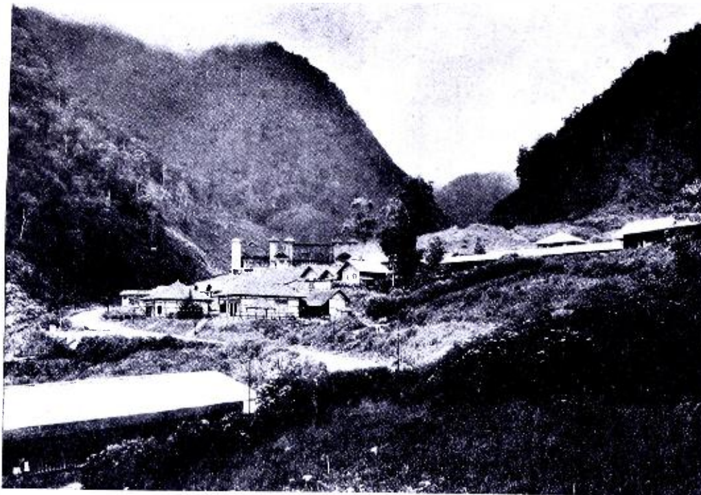
MALABAR TRANSMITTING STATION NEAR BANDOENG, JAVA The vertical fan antenna is strung between two mountain peaks!
