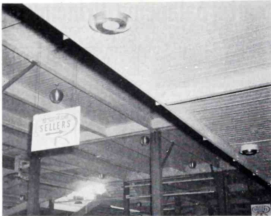
FIG. 2: SPHERICAL BAFFLES suspended from unfinished ceiling at left and flat fixtures at right are employed in areas where flush ceiling mounting could not be utilized. Both types of fixtures were designed by Soundolier and contain Jensen speakers.
