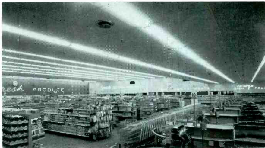
SOUND SYSTEM for a super-market using ceiling speakers and check-stand units designed and installed by Electrical Communications.
