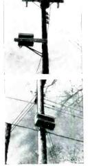
Two views of SKL Model 212TV Amplifier mounted in Model 420 Amplifier Cabinet, mounted on a telephone pole crossarm (top), pole (bottom). Courtesy Vermont Television, Inc.
