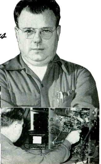
2. LOCATING THE SHORT—With Loadchek you can quickly check the shorted side, part by part, without laying down tools or picking up test leads. Here, the trouble was a short in the transformer, spotted without having to warm up set. Overloads are found the same way.
