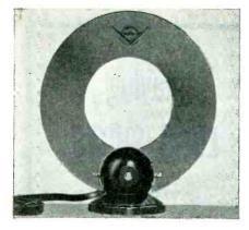
Indeor uhf full-wave flat-loop antenna. Model is ten inches high and nine inches wide, and weighs under a pound. The loop is of rose goldcolored anodized aluminum, with a mahogany phenolic base which is weighted to prevent tipping. (Buliseye; Radion Corp.)
