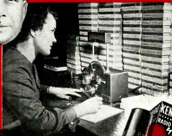
WALTER DOWNING , Foreman, Raw Materials Inspection Department, is in charge of comprehensive testing of all materials used in making Ken-Rad tubes. Here cathode sleeves are being tested for breaking strength.
