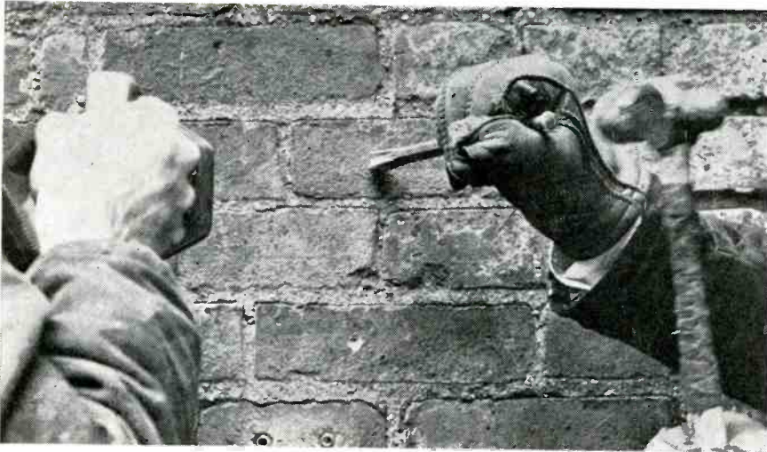
Fig. 3. At left, appears a hole being made with an electric drill, and at right, a hole being made with a star drill and hammer.
