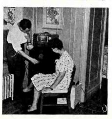
Rotating an f-m dipole for maximum signal response.
