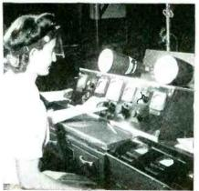
space, and beneath a drawer for paper, forms, pencils and so on. On either side of the writing space are more meters. Where the desk drawers would be there are switches and controls for the power supply which forms part of the test position and which provides all required voltages for the widest array of cathode-ray tube types.
