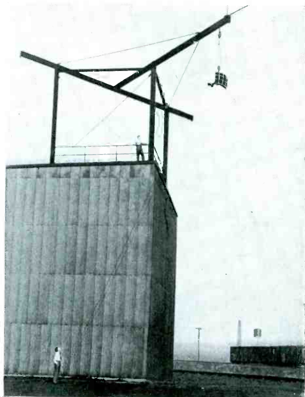
Fig. 6. Ranging among the largest of similar structures, Jensen's new soundroom is nearing completion. According to Hugh S. Knowles, vice-president and chief engineer, the new soundroom will permit a more accurate determination of the response and directional characteristics of loudspeakers at low frequencies and will greatly facilitate precision acoustical measurements. Rigging is also provided for outdoor measurements as shown in the photograph where the performance of one of the new Jensen 60-cell type "K" Horns, equipped with 2 type X permanent magnet driver units, is being determined.
