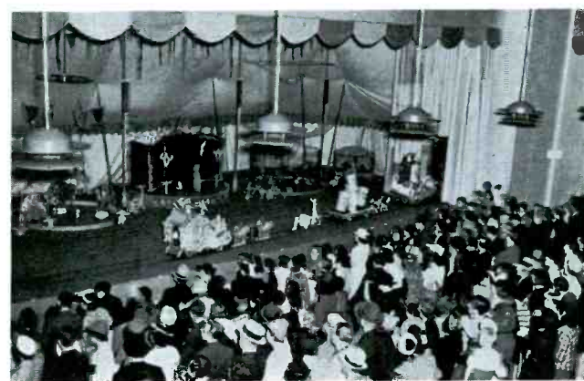
Fig. 11. Sound is localized in the installations at the Beechnut exhibits by projecting it directly down from overhead. Two methods of supporting the speakers are used, one in a canopy-like baffle (shown below), the other in individual decorative metal housings suspended from the ceiling (shown above). An Operadio amplifier with Garrard automatic record players are employed in each case.
