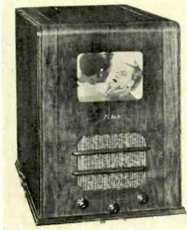
G.E. HM275 (below) combines an all-wave radio with a television receiver. It employs 29 tubes and a 12-inch kinescope.
