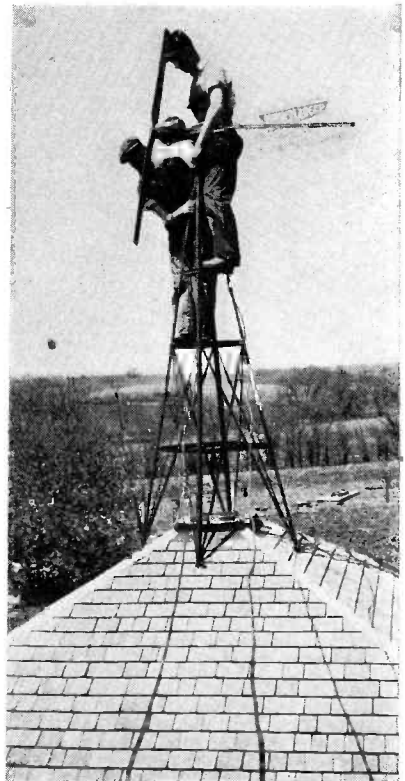
Two farm boys take time out from chores to install a wind-power charger. This illustrates a typical installation as recommended for flat country.
