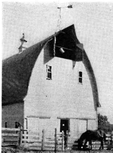
An Iowa barn serves for this mounting.
