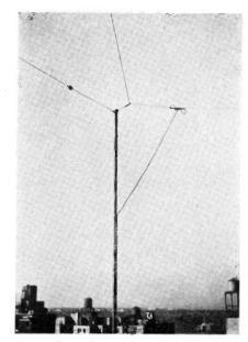
Fig. 2. Typical iron-pipe mast for master antenna system.
