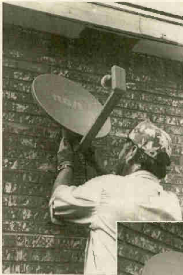
The 18" dish can be installed on a south-facing wall by the user or by professionals. David Hutson of Baillio's Warehouse Showroom intalls this one at a home south of Albuquerque. How is this for a replacement of the huge dish you may now own? Photos by B. W. Battin.
