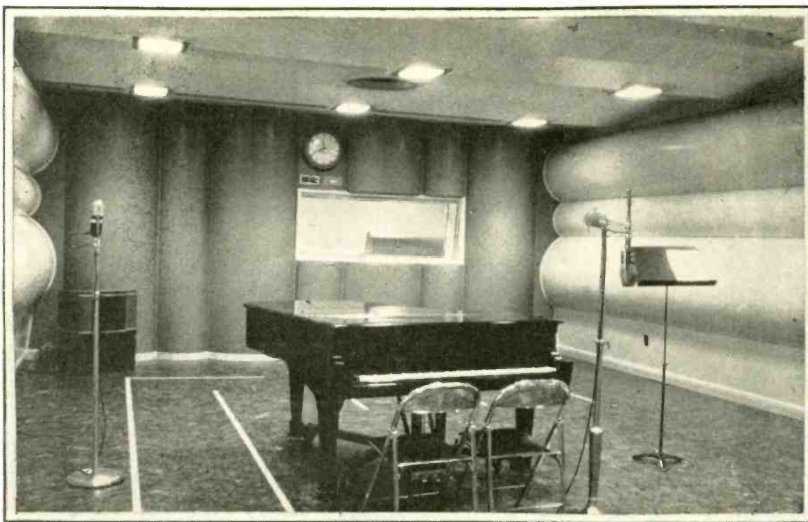
Fig. 1. The comparative improvement of the convex-panel structure over the conventional parallel-plane wall studio in beauty as well as operation, is illustrated in this view of Studio "C", WFAA, Dallas, Texas
