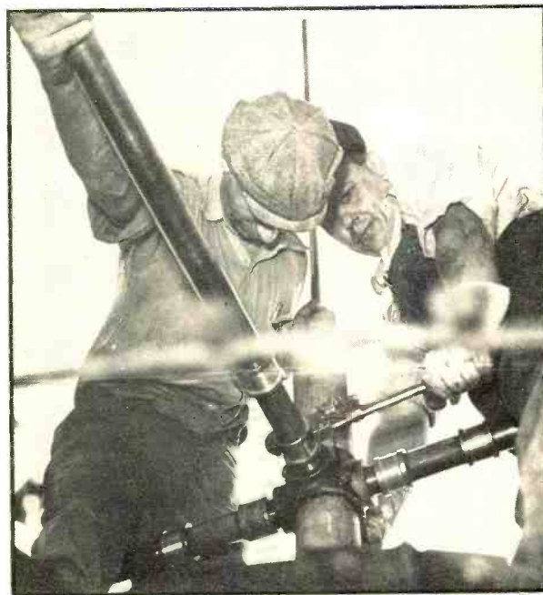
The last of the upper bay radiator elements is fitted into place. Lightning rod rises 5 feet above top of 4-inch supporting pipe. Micarta insulators show at inner ends of radiator elements.
