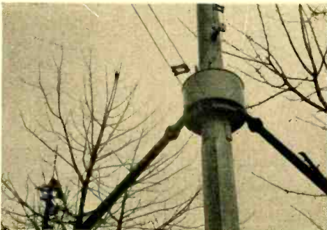
The slip-ring feed system shown with its protective cover.
