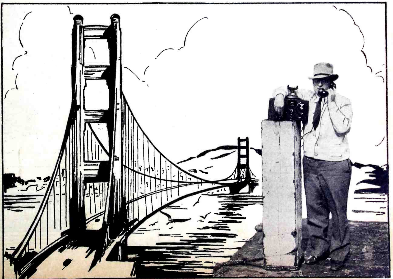
5-Meter Portable Radiotelephone, An Aid to the Bridge Builder. See Page 16.
