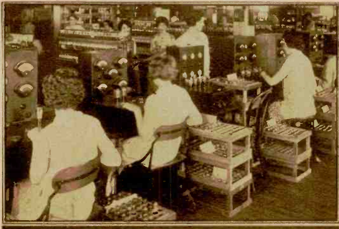
(Left) Factory Testing of Hygrade Tubes
