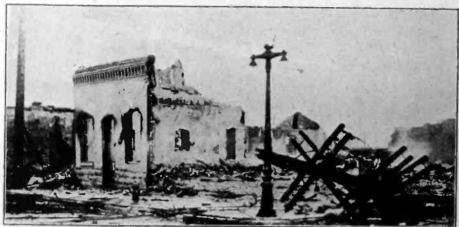
Electrically Transmitted Picture of Tornado Damage at Murphysboro, Ill.
