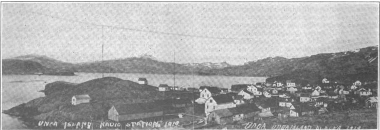
Commercial radio station at Unga, Unga Island, Alaska (KVI), constructed by the author. In this picturesque village of the "Samuel Jones" stories, something of the untamed spirit of earlier Alaskan days is still discoverable.
