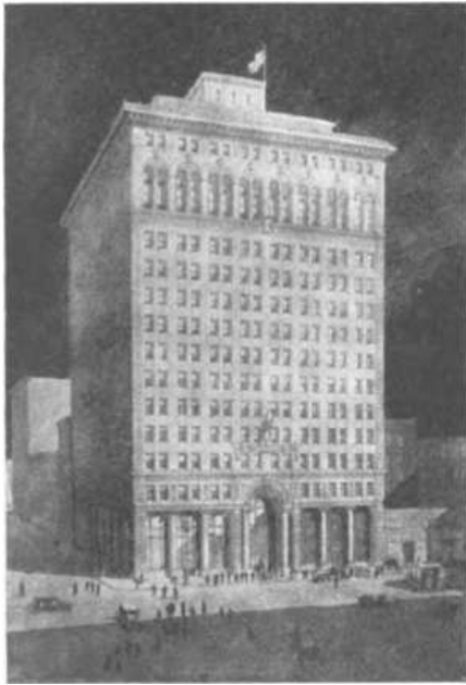
Matson Navigation Co. New Building to be wired for Radio.
