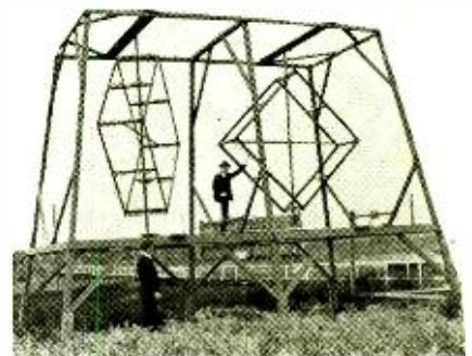
A 5,000 mile aerial! These loops are used for receiving. By means of gears and shafting the loops can be rotated by the operator at his desk (Kolster loop circuit). would be from the windmill,” said Bill, disgruntled.
