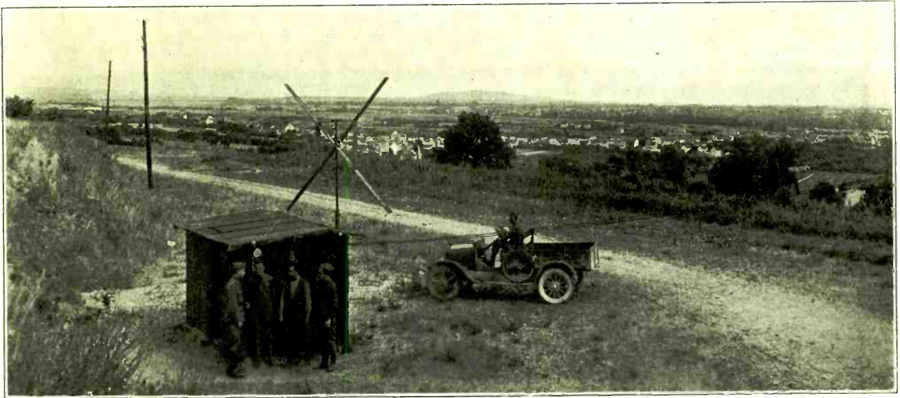
Signal Corps Continuous Wave Station Twenty Miles West of Paris After the Armistice to Communicate With Spa, Coblenz, Treves, Antwerp and American General Headquarters Replacing Telegraph Lines Which Were Turned Over to French. As High as Eight Thousand Words Were Handled by This Station in a Day. Note the Loop for Reception to Eliminate Interference.
