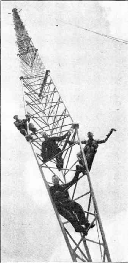
Steel riggers about to start their daily climb to the top of KDKA's vertical antenna during the course of its construction. Now completed, it is 710 feet high and weighs 60 tons.
