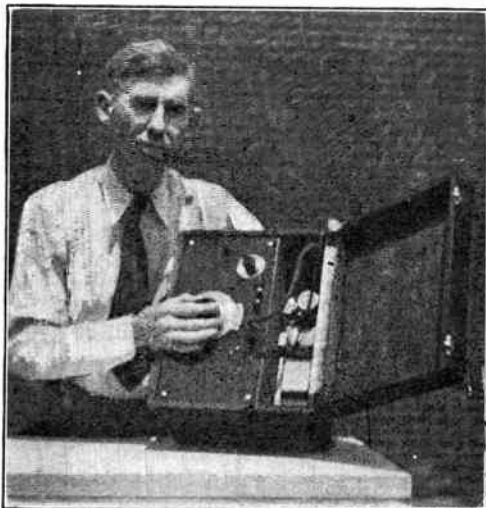
The oscillator and amplifier fit nicely into a wooden box. The author is manipulating the dial.
