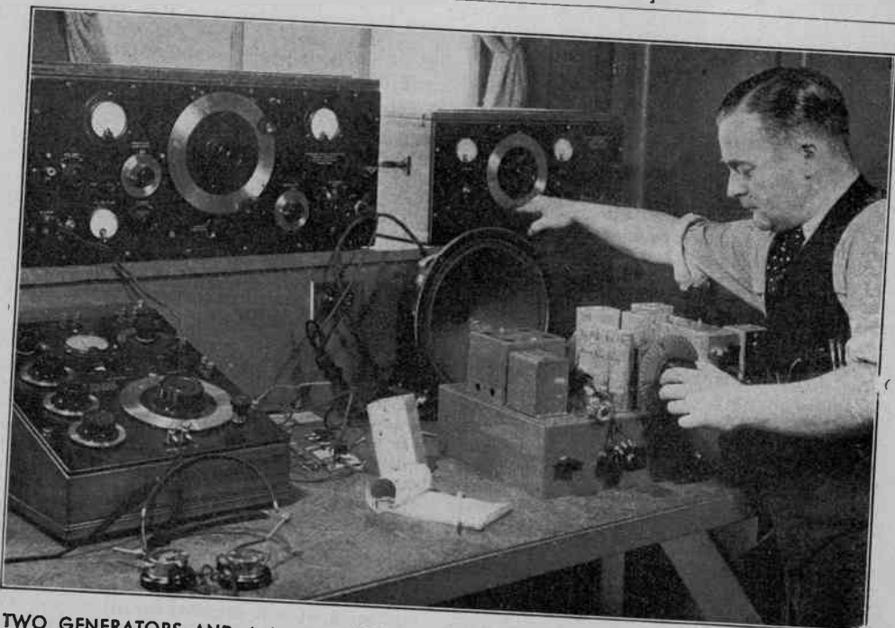
TWO GENERATORS AND A BRIDGE ARE AMONG EQUIPMENT USED IN MEASURING AND ALIGNING NATIONAL COMPANY NC-100 RECEIVERS.
