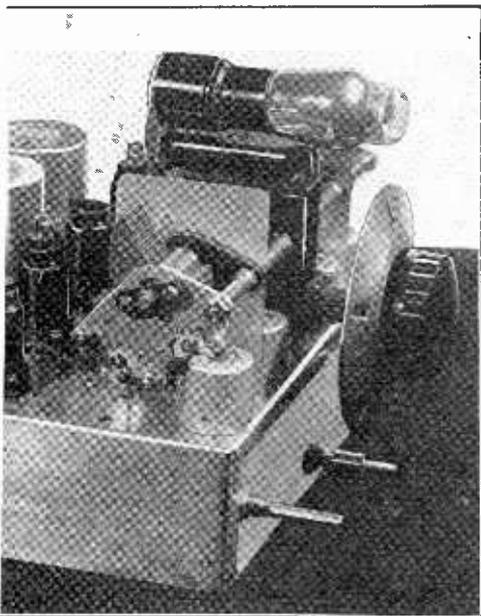
rear, close to the pair of electrolytic condensers. National PW-4 tuning unit is the so-called "magic" tube the 6E5, this tube is of the cathode ray indicator type. The angle denotes resonance.
