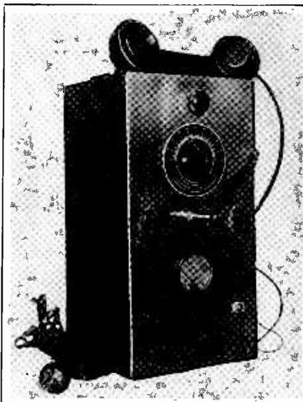
The French type earphones are plugged into a front panel jack when the dual switch is at "Receive" position.
