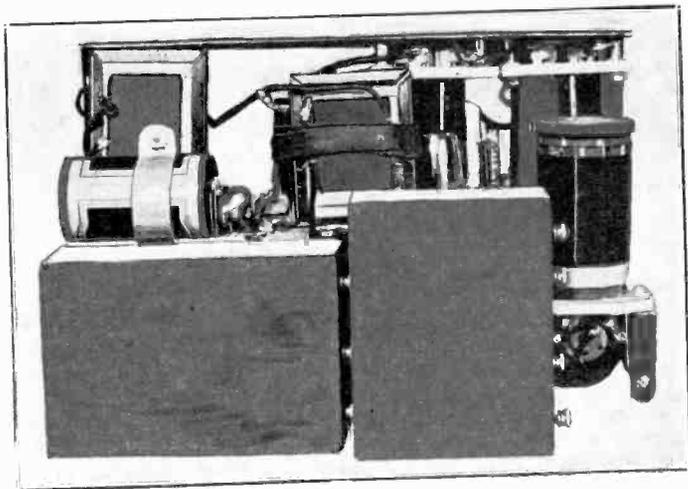
Battery sets should be carefully tested for polarities, as it is easy (oh, so easy) to incinerate the filaments by misapplication of potentials. Be sure, by continuity test, that the B plus post of the set reads as if an open to the filament, before batteries are connected.
