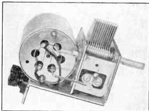
A wave trap is very effective in cutting out an interfering station, but the coupling to the remedied circuit must be very loose.
