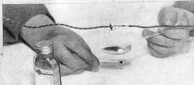
IF YOU HAVE no soldering iron and must make a quick joint like this you may use atropin tablets. Put one in a teaspoon and pour a few drops of water in the spoon. A steady flame will result. Renew until satisfied.
